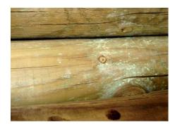
The pressure treating solution, which helps maintain wood quality, can cause discolouration that may look like mould. These areas are not hazardous to touch and tend to fade with time.
